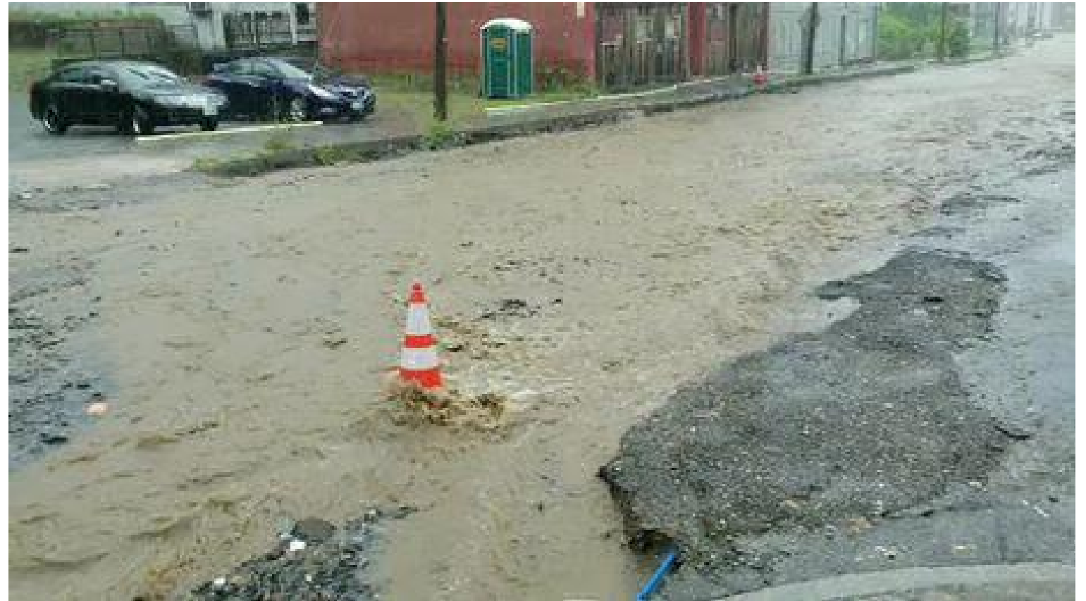
A muddy mess poured down Main St. following torrential rains on Friday and Saturday, eating away at the exposed dirt and broken up pavement (Courtesy photo).
