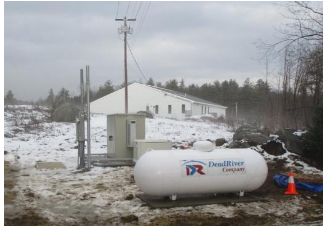
The metering station, where service branches out to the other parts of town. The source of internet comes from Manchester via a fiber optic cable routed through Keene.
