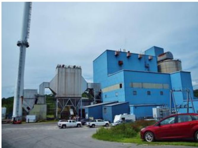
Springfield Power in Springfield, NH, was one of the state's six independent biomass energy plants and a vital market for low-grade wood and wood chips. (Photo by NHTOA).
