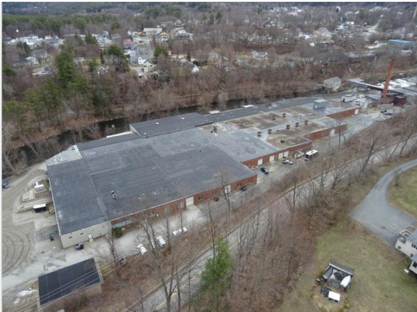
The large multi-business commercial building at 247 Sullivan Street (Courtesy, State Attorney General’s Office).
