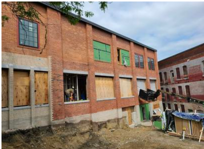
Views from opposite directions. Once the granite window sills were installed, the openings were readied for installation of large, energy-efficient windows. Meanwhile, rooms on the first floor are at the frame-out stage; sheet rock walls are soon to follow (Eric Zengota photos).
