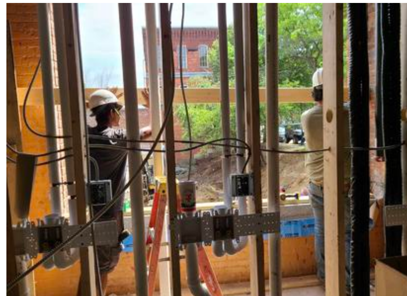
Views from opposite directions. Once the granite window sills were installed, the openings were readied for installation of large, energy-efficient windows. Meanwhile, rooms on the first floor are at the frame-out stage; sheet rock walls are soon to follow (Eric Zengota photos).
