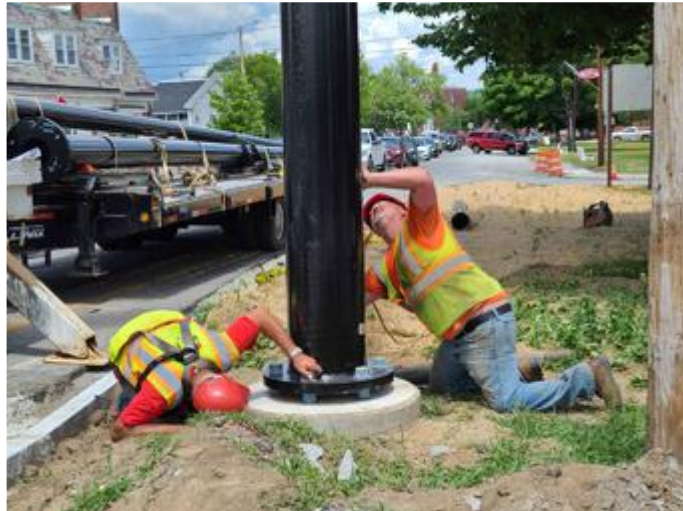
Top left and center: Tri-State Curb is in charge of sidewalk installation. Right: New England Signal Systems workers hoisted the 35-foot pole for the permanent traffic signal on Broad Street, then positioned and slotted it, finally tightening the bolts to secure it to the slab. The new traffic signal will replace the temporary ones currently hanging over the Broad and Glidden intersection (Eric Zengota photos).
