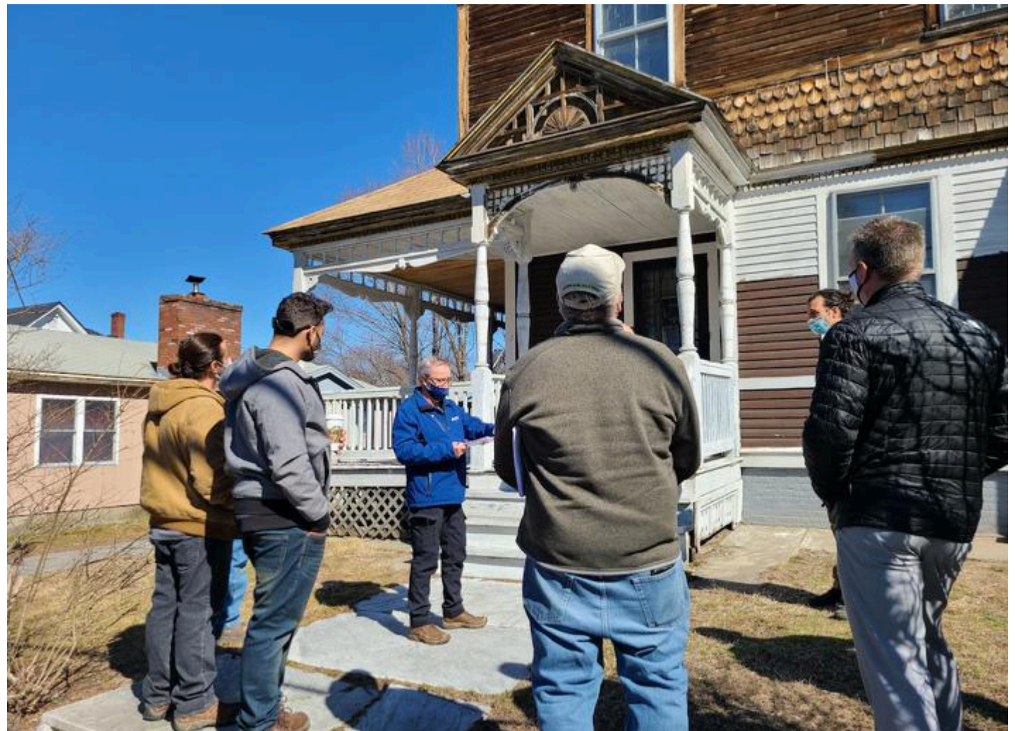
Mickey Laskey (center) points out which parts of the exterior of 31 Myrtle Street need remediation (Eric Zengota photo).
