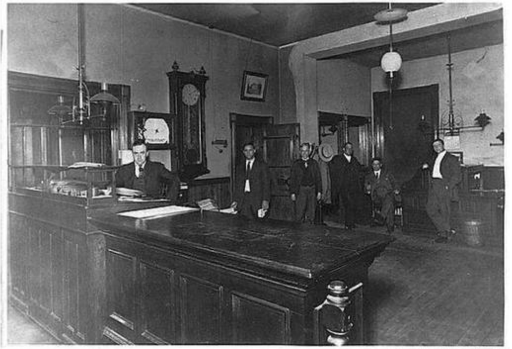
Claremont City Hall office, in the early 1900s (Photo courtesy of Joseph Rzczycki).
